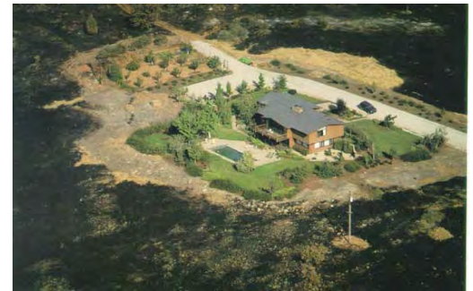
While the fire burned all around, defensible space, gave firefighters the chance to save this home.
